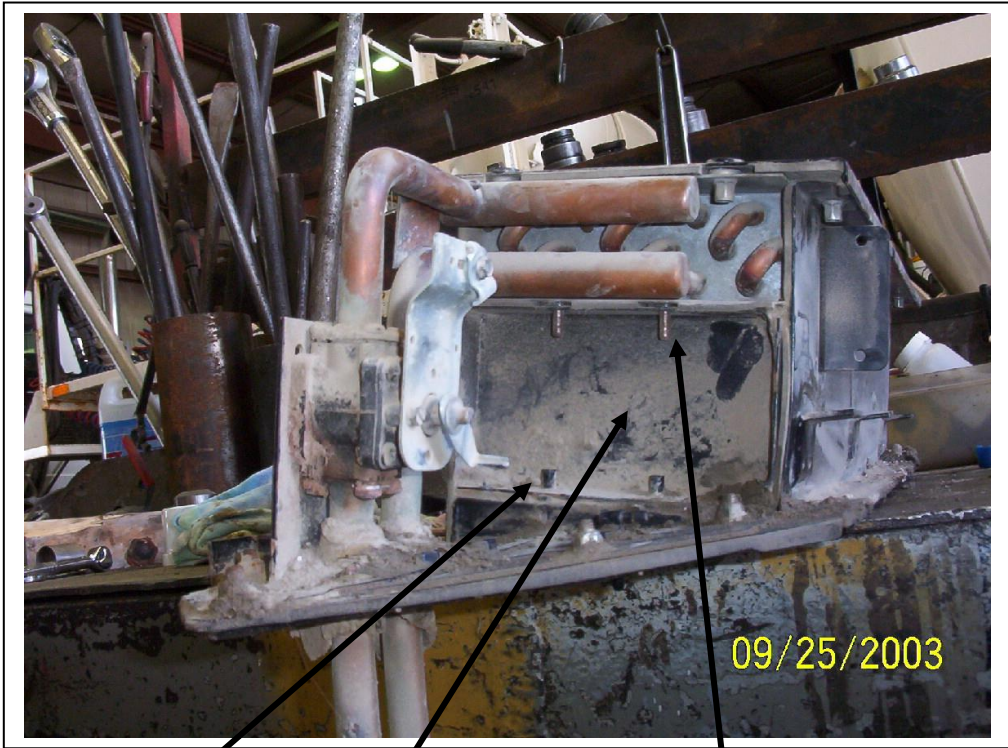
Locator pins on heater coil
