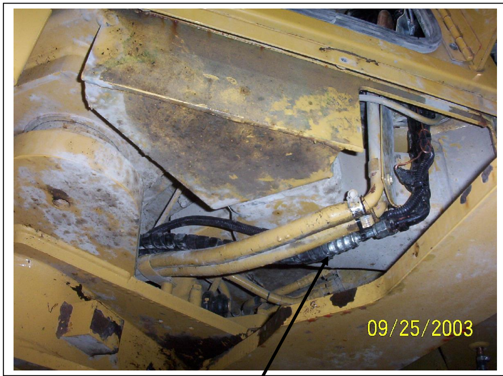
A/C hoses connected and secured to heater lines.
